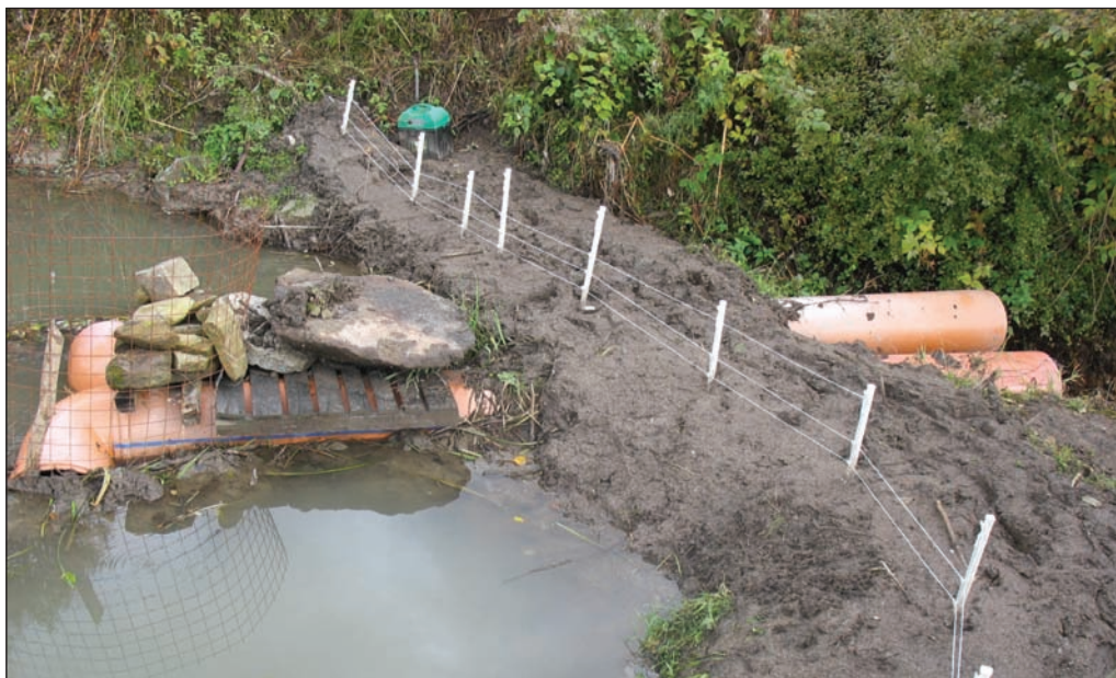
Figure 21. Culverts placed through a beaver dam in Bavaria lower the water level in the pool behind it. The left-hand end of the culvert incorporates an angled section of pipe that can be turned to raise or lower the water level. The electric fencing along the top of the dam is temporary to deter further dam creation downstream. The bare earth will grass over during the coming spring. The total cost for materials was less than €250.
