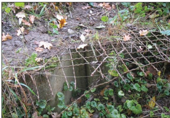
Figure 20. Embedded metal piling and wire grids protect flood embankments on the Danube from animal burrowing, including from beavers.
