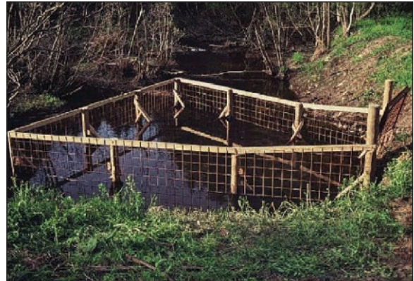
Figure 19. Post, wire and corrugated metal constructions are very effective at protecting culverts from beaver activity. They are relatively inexpensive and easy to install. S. Lisle, S. Tippie.
