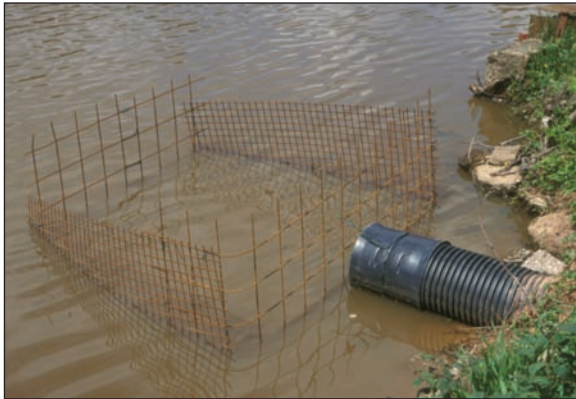
Figure 19. Post, wire and corrugated metal constructions are very effective at protecting culverts from beaver activity. They are relatively inexpensive and easy to install. S. Lisle, S. Tippie.
