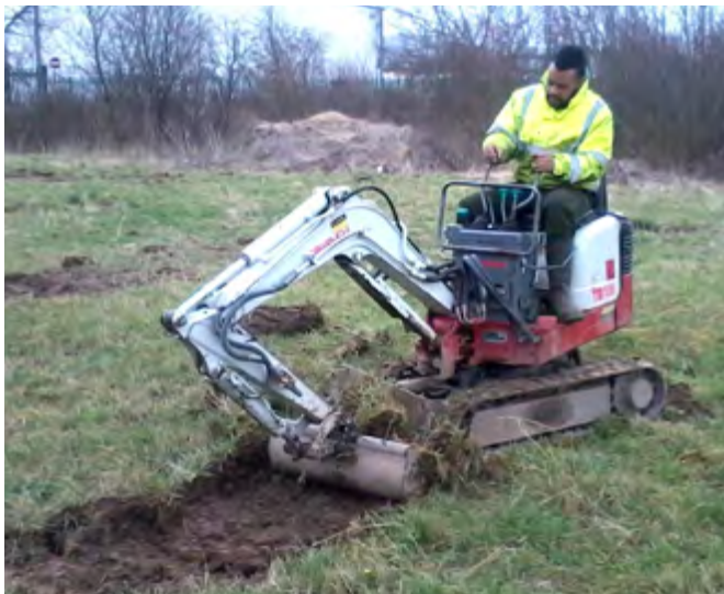
Topsoil stripping with mini-digger
